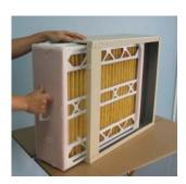
7. Re-install assembly into the main air cleaner housing. Replace the access door.
